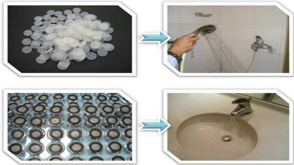
**Figure 3.0 Installation of Water – saving Restrictors on the Taps and Showers of the Hospital**
