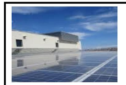
The 108 solar panels stretched over an area of 190m<sup>2</sup>. It generates electricity during sunshine hours and feeds into the electricity grid. At night it goes into standby mode. This system does not export power into the municipality grid therefore Khayelitsha hospital is a net
